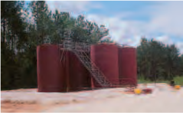
New tank facility at Shoats Creek
