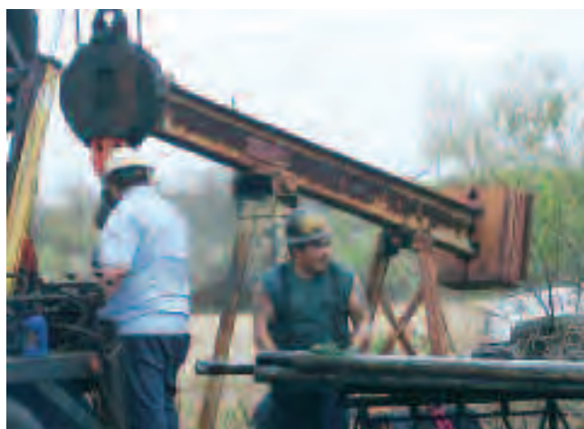
Well workover at Somerset
