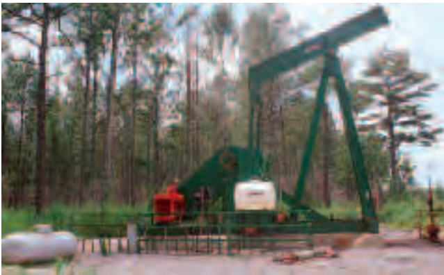
Installing new pump at LM#9, Shoats Creek
