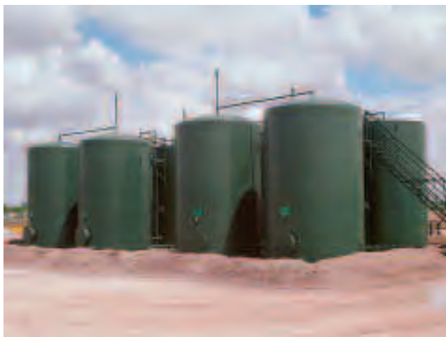
Tank battery at South Weslaco
